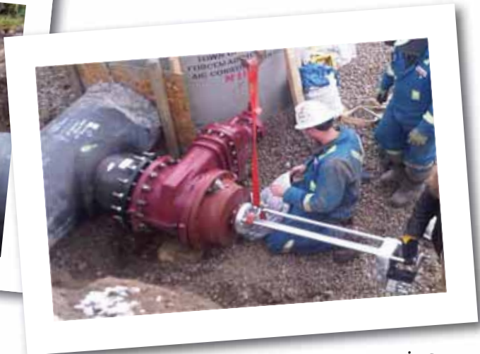
Canada - 28"x14" IPS EF saddle hot tapping application
