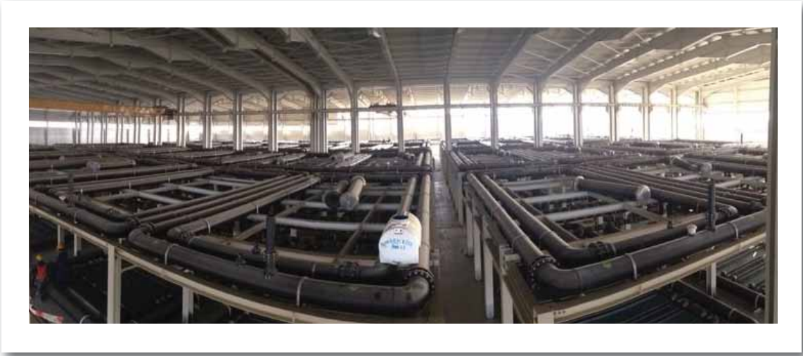
Azerbaijan - Bakü Infiltration - Water treatment plant 3700 EF Saddle and 19,500 fittings connection
